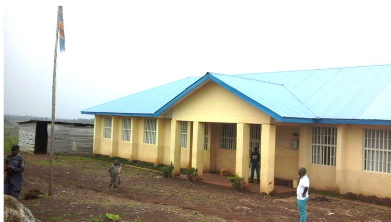
Figure 1: This is the main police station in Kavumu where only two police officers are permanently placed. In case of an attack or as a response to a distress call from the village there is no troops to intervene.
